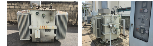
Before Replacement (Aging Transformer)
